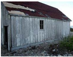
Boat house roof
